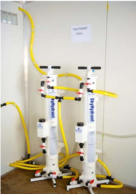
The SkyHydrant consists of thousands of micro-porous hollow fibers. Through pressure created by flowing water, turbidity and any solids as well as germs like bacteria, protozoa or pathogens, which have lower molecular weight than water, are removed while water molecules pass through the membrane. No chemicals are required for the filtration process hence the water is pure and safe.
